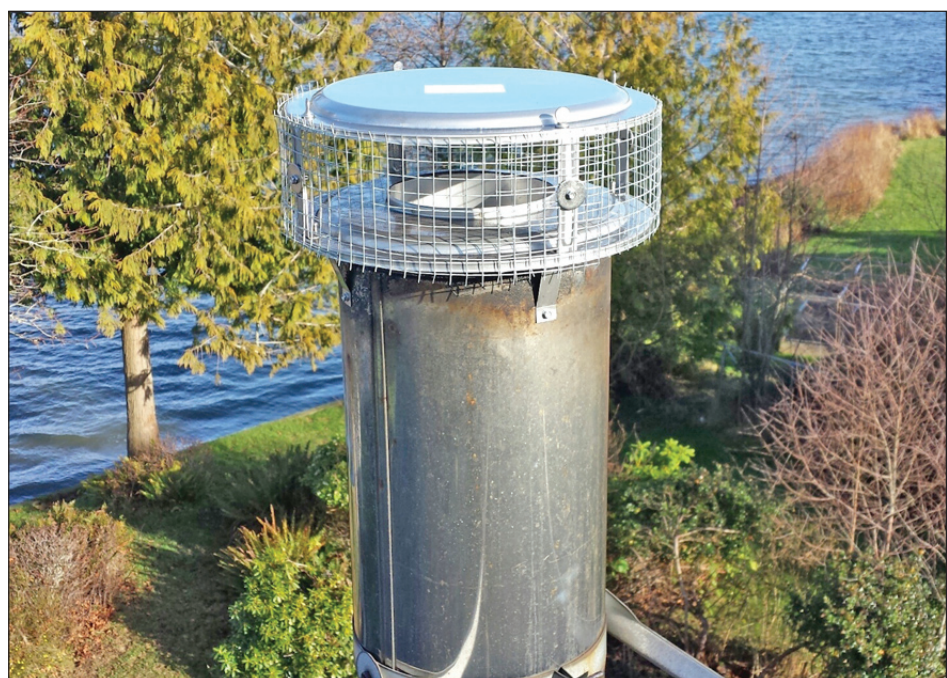
Chimney caps and spark arresters, pictured here, not only can help keep the wild critters out but are crucial fire safety devices as well.
